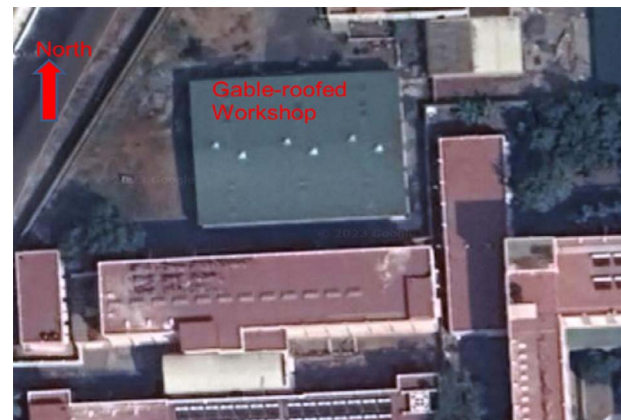
Figure 16. Satellite image of workshop complex.
