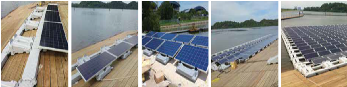
Figure 10. The construction process of FPV systems on a water source [17].
