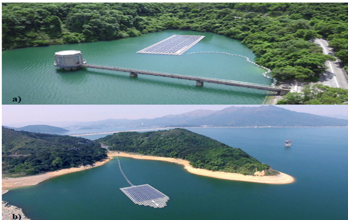
Figure 12. 100 kW FPV power plants located at (a) Shek Pik and (b) Plover Cove reservoirs [39].
