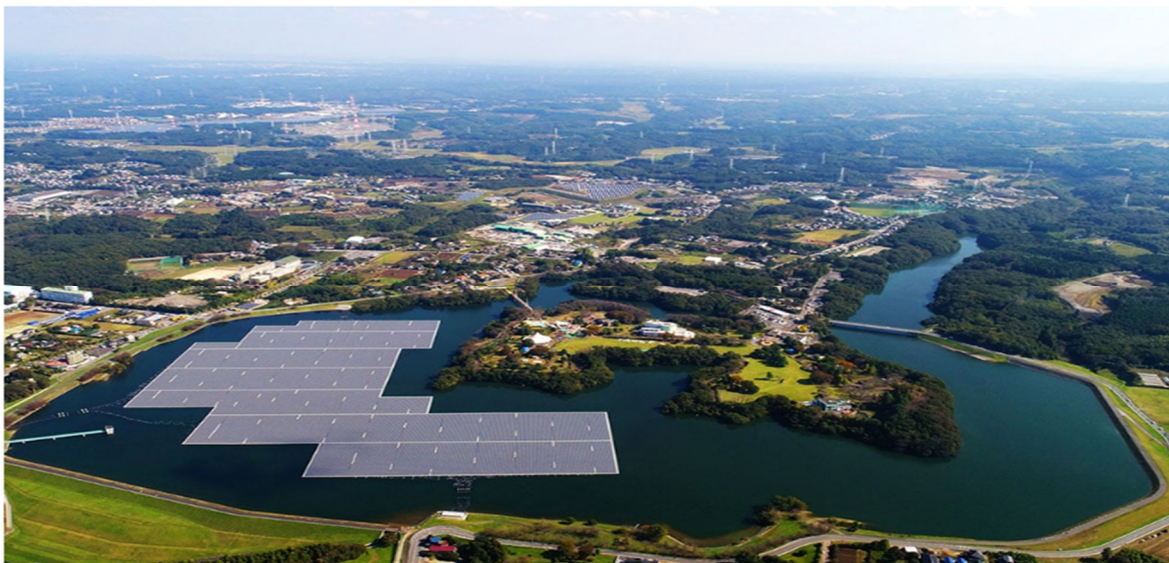
Figure 9. Land-saving by large-scale FPV installation covering the water surface in Japan [20].
